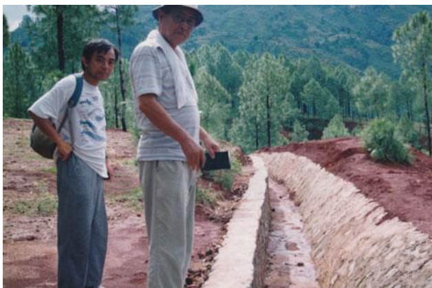
Fig. 7 Catch drain for diversion of run-off water from the Upper Slopes
