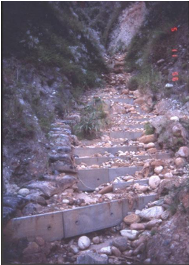
Fig. 6 PNC plates installed on the gully bed of RB4
