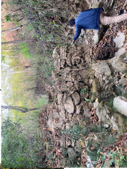
Check dams has been remaining though partial damages Dahachowk (2024.4)
