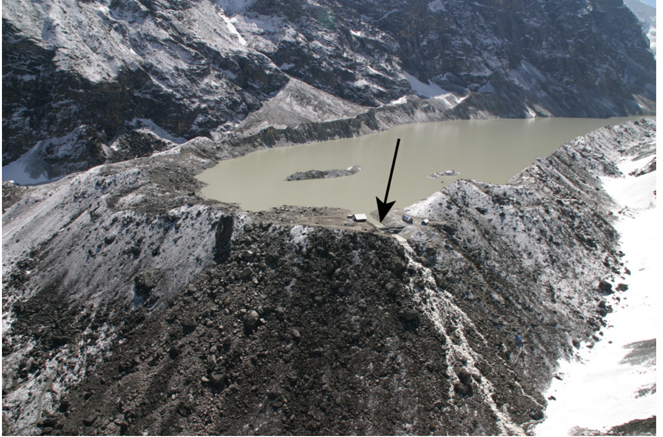
Figure 22. Photograph showing eastward view of the terminal moraine forming Tsho Rolpa glacial lake. The engineering outlet works (fig. 23) are indicated by an arrow.
