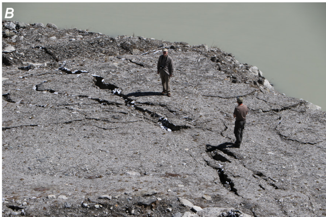
Figure 24. Photographs showing lateral spreading at the inlet to the Tsho Rolpa engineered drainage channel (A, B). Approximately 1.0–1.5 m of horizontal displacement (toward the lake) and 0.5 m of downward displacement on the eastern side of the channel did not appear to compromise the stability of the moraine dam or engineered outlet.
