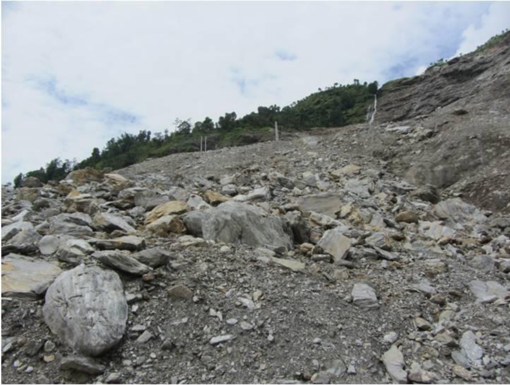
Figure 12: Debris deposited at the toe part of the Landslide
