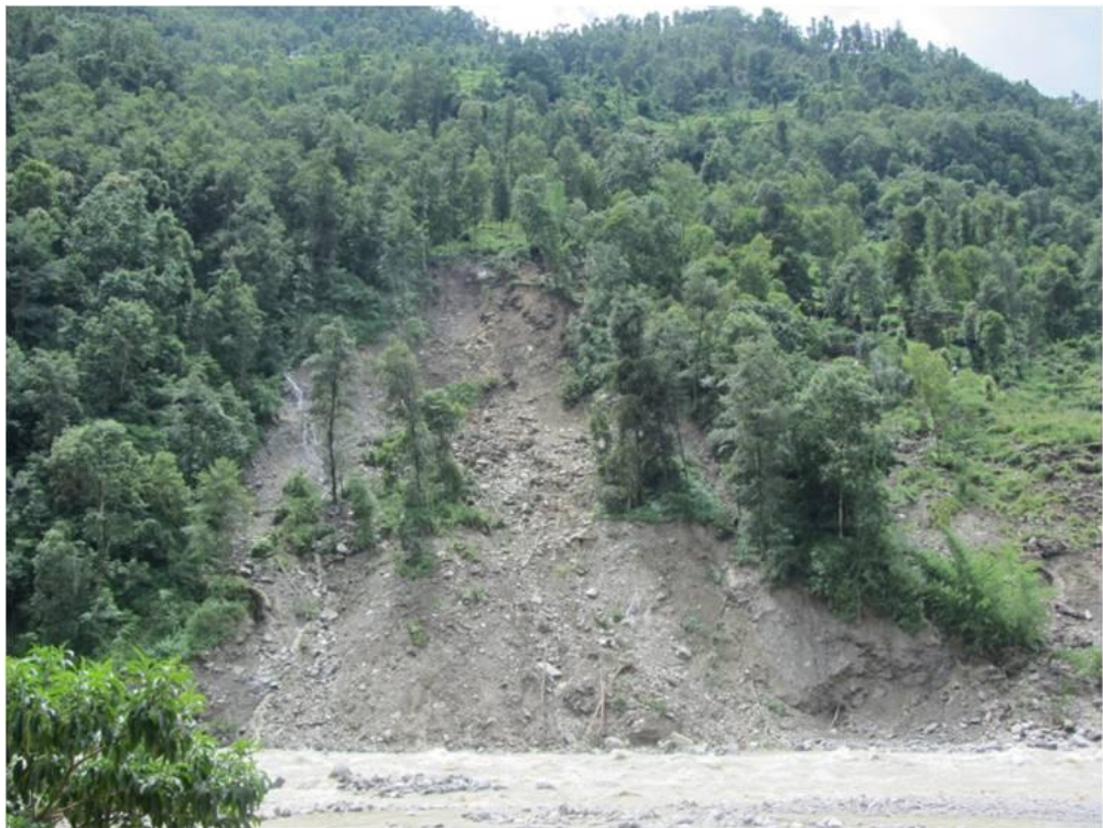
Photo 6: Landslide occurred at left bank of Sunkoshi after breach of Dam
