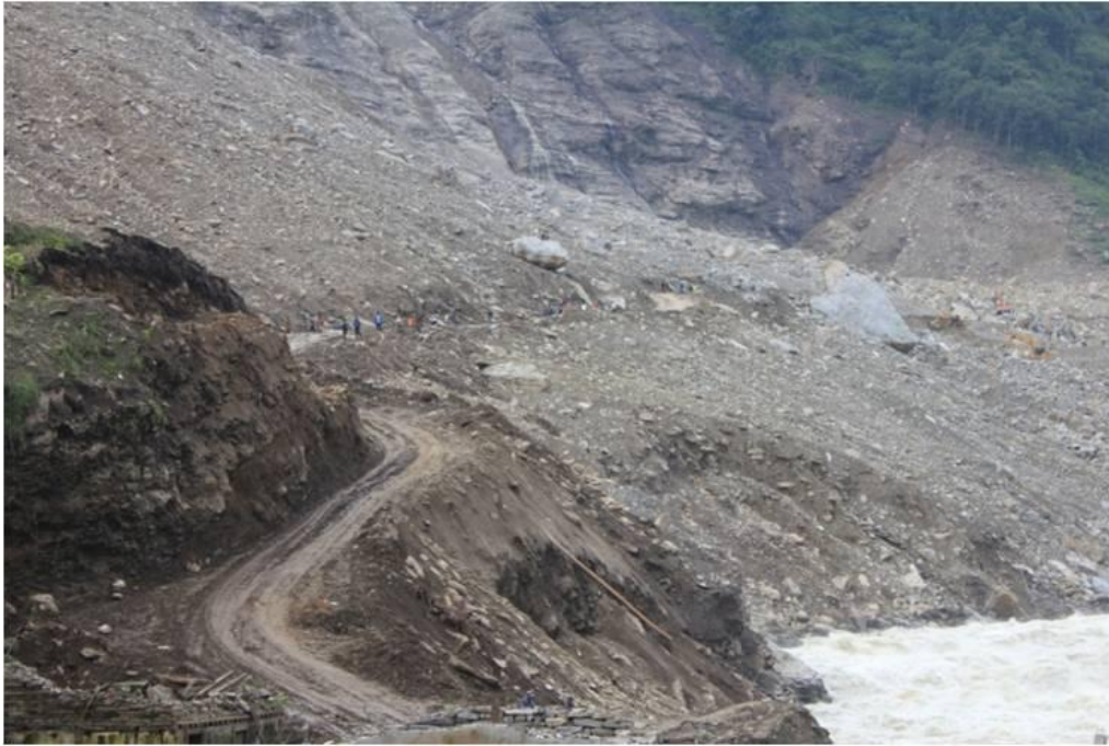
Photo 1: Temporary Araniko Highway track at toe of the Landslide
