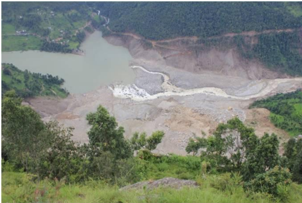
Figure 13: Opening of Secondary Channel in the Landslide Dam
