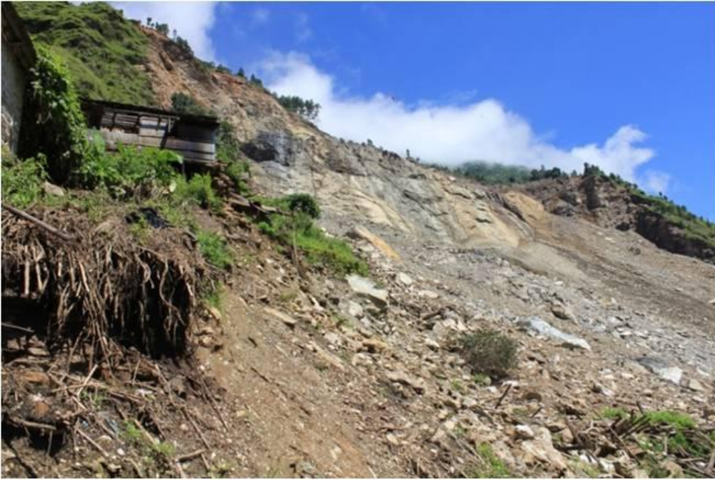
Figure 9: Landslide near the damaged village Iteni
