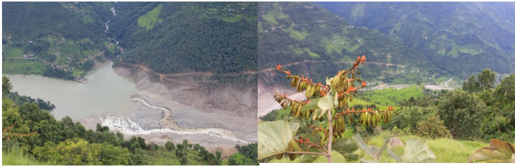
Figure 15: The alternate temporary road to Barahbise constructing by Nepal Army
