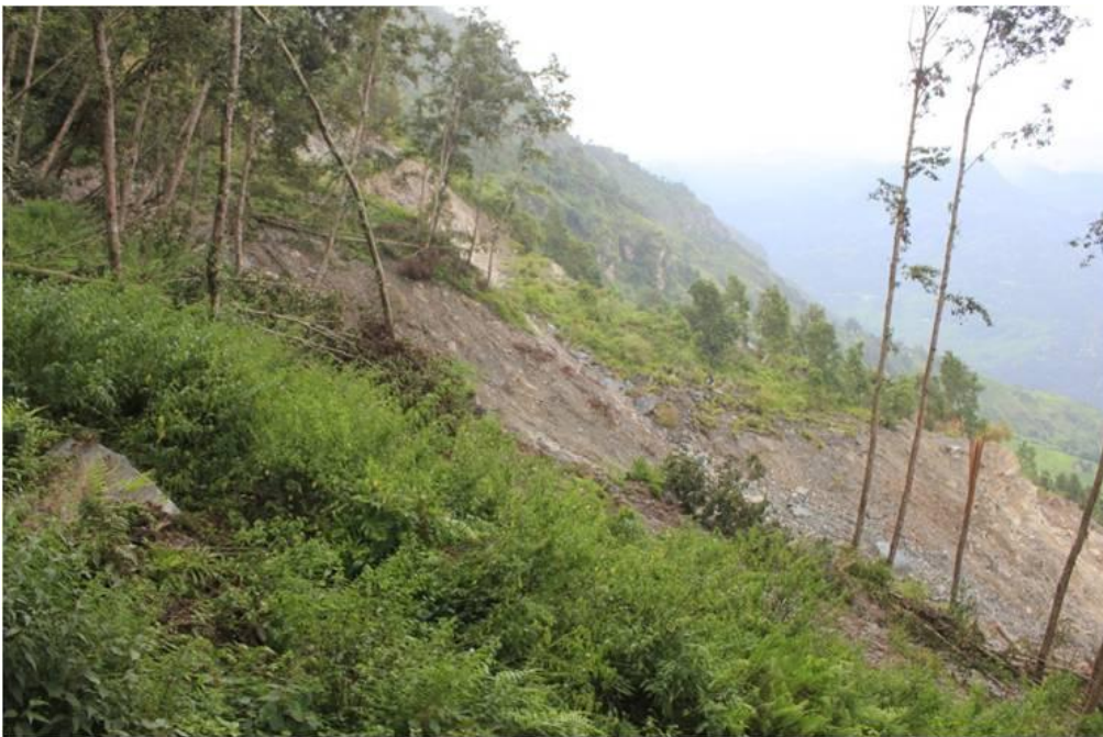
Figure 2: Cracks and disturbed surface in the Crown part of the Jure Landslide
