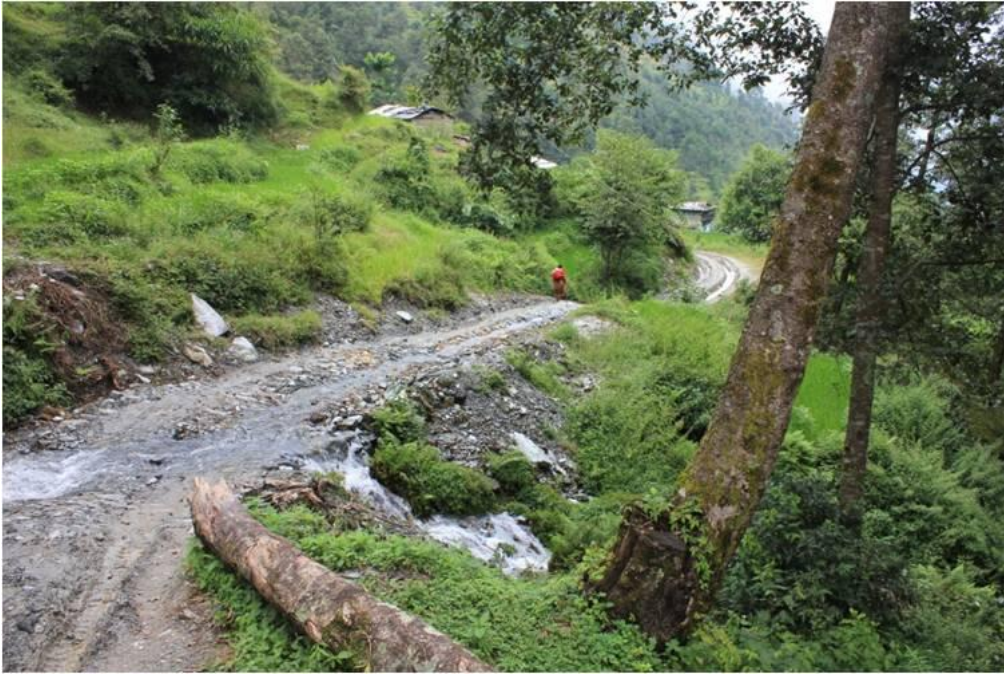
Figure 5: Subsided village road in the crown part of the Landslide
