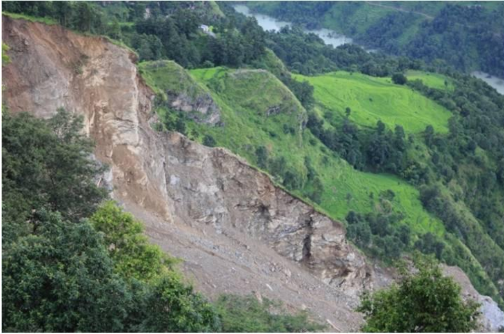
Figure 8: Big cracks near the border of Landslide
