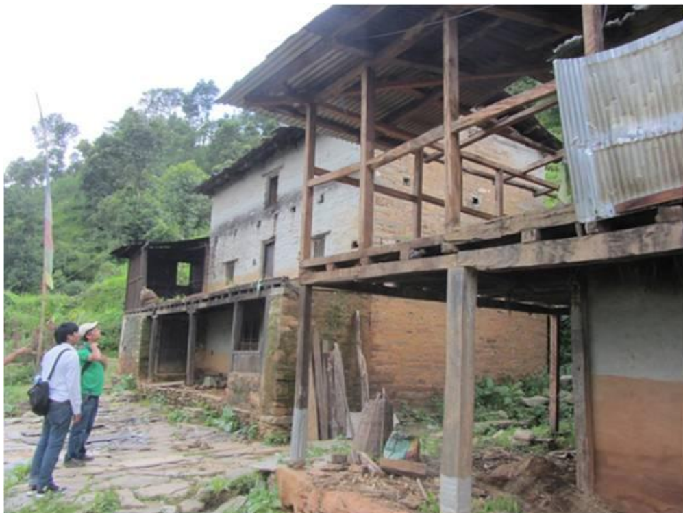
Photo 4: Damaged houses due to the Landslide
