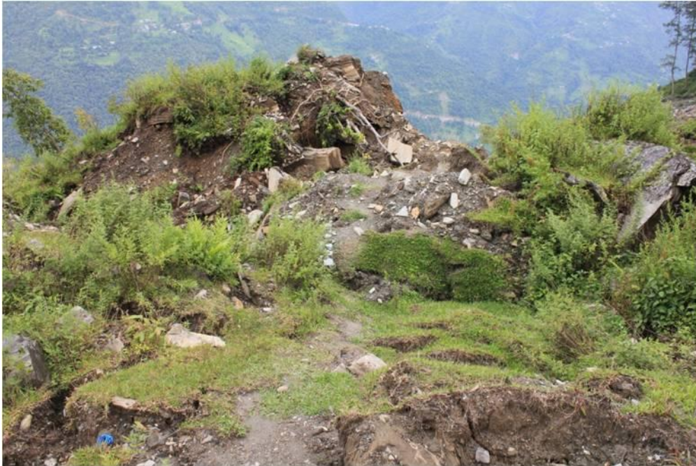
Figure4: Cracks and ready to move mass in the Crown part of the Landslide
