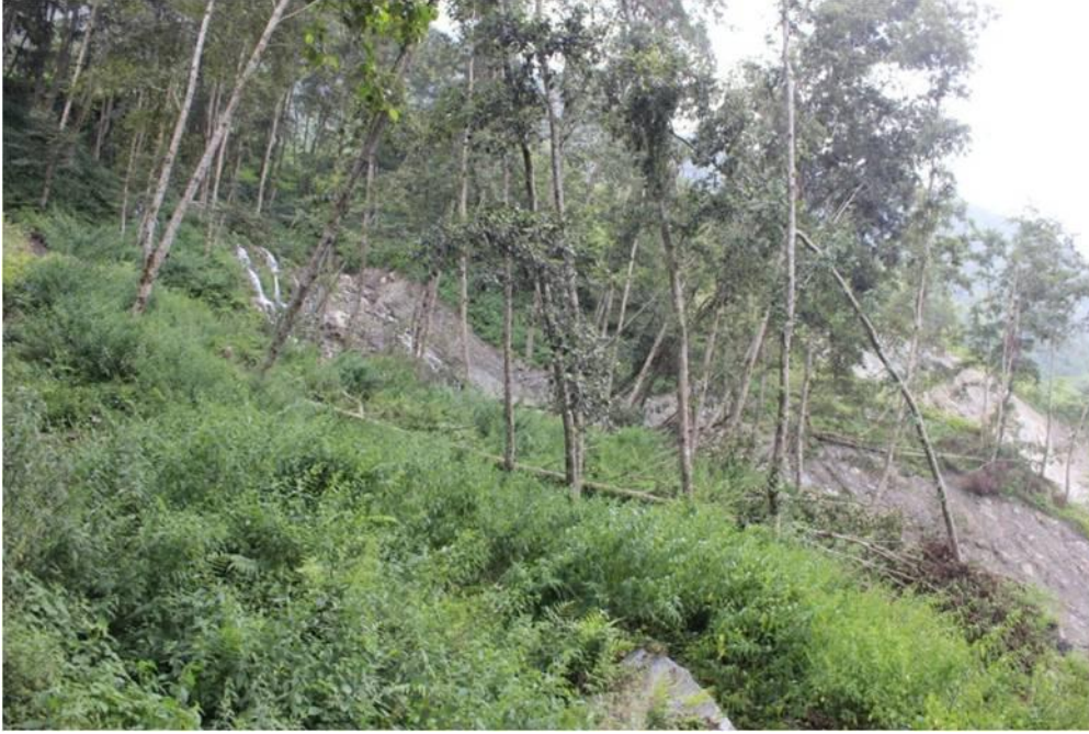
Figure 3: Disturbed and inclined trees in the crown part of the Landslide
