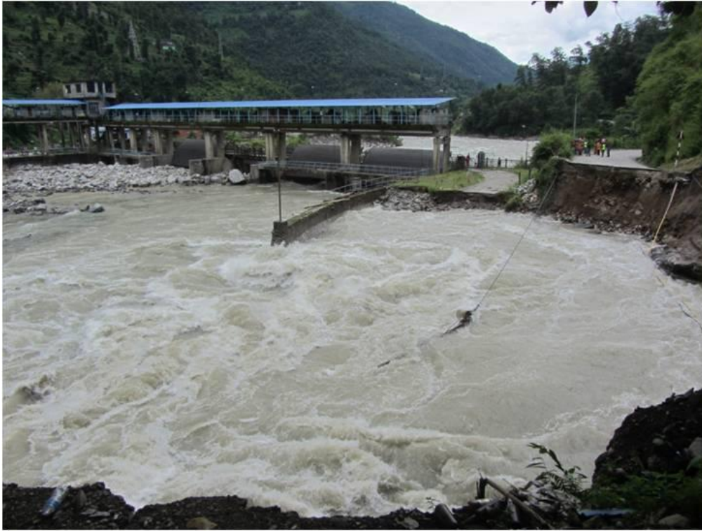
Figure 14: Damaged Sunkosi Hydropower Headwork and Araniko Highway after breach of the Landslide Dam
