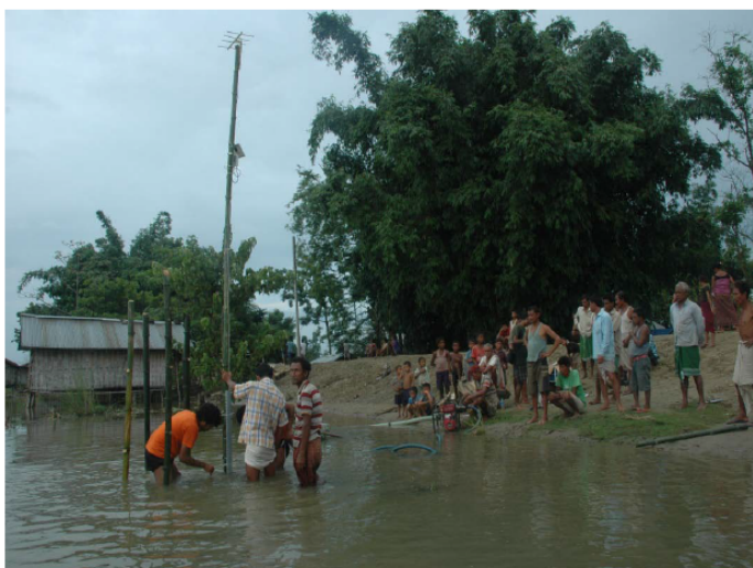
Flood early warning system installation at Dihiri along Jiadhah River (Dhemaji District). Credit: ICIMOD
