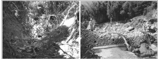
Fig. 1. Example of masonry check dams in Hiroshima Prefecture damaged by heavy rain in July 2018.
