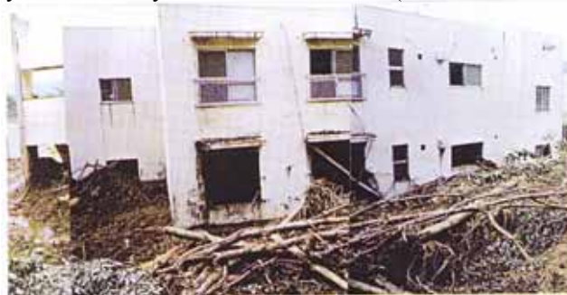
Photo-2 A debris flow that occurred at a hill behind a social welfare facility directly hit the facility, claiming 5 lives (Fukushima Prefecture). (August 27, 1998)
