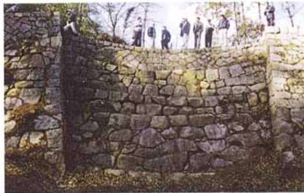
Photo-1 Fukami sand retaining works – This dam was constructed by stone masonry in Dodo River in 1854 (Hisoshima Prefecture)
