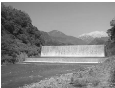
Fig. 1 Hongu Sabo Dam
