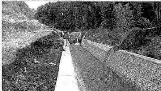
Photo 2 The upstream section of channel work
