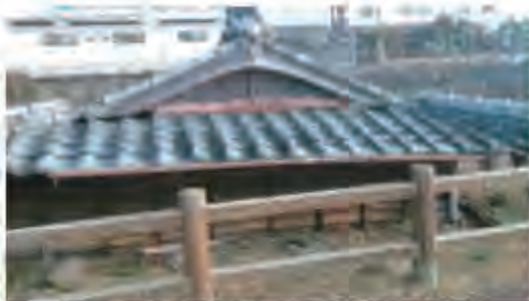
Figure 22 Buried House at Memorial Park
