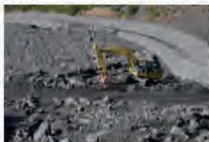
Figure 9 Unmanned Heavy Equipment to remove debris deposit
