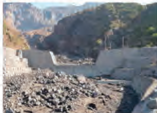
Figure 12 Sabo Dam no. 8
