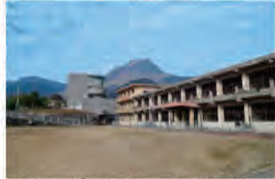
Figure 29 Ōnokoba Elementary School burned by Pyroclastic Surge
