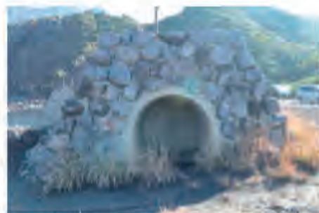
Figure 15 Emergency Shelter at Sabo Dam Structure
