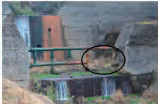
Figure 18 Open Type Sabo Dam
