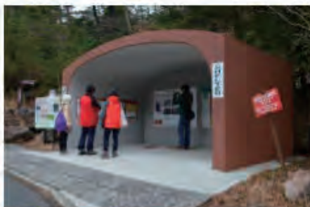
Figure 4 Emergency Shelter at the Entrance of Onaminake Lake Track
