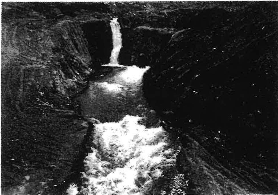
Figure 11. Completed Downstream Portal During Lake Drawdown Period
