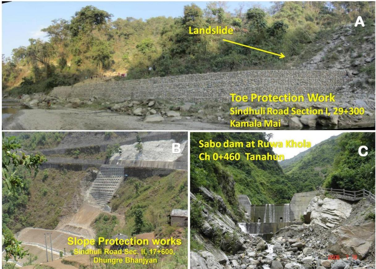
Figure 10. Landslide mitigation measures implemented in Nepal. A) Toe protection works to mitigate slow moving landslide, Sindhuli Road, Section I, 29+300m (Amatya & Mori, 2018), B) Slope protection works by anchoring to mitigate slope failure, Sindhuli Road, Section II, 17+600, (Amatya, 2016), C) Debris flow mitigation works by Sabo dam, Ruwa Khola, Marshyangdi Hydropower, 0+460, Tanahun (Pandit, 2009).
