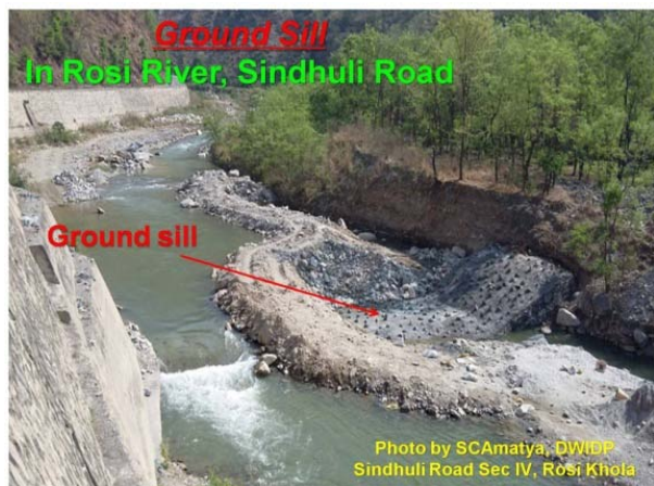
Figure 2.10: River Bank protection with construction of Ground sill, Sindhuli road, sec IV, Rosi Khola
