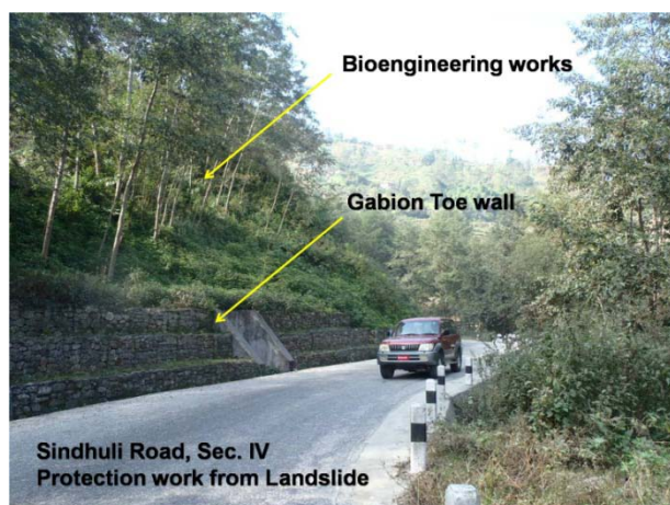
Figure 2.11: Road protection from landslide by construction of gabion toe wall and bioengineering works, Sindhuli Road, Sec. IV.
