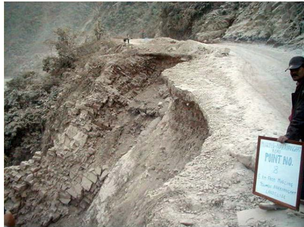
Figure 1.5: Damage of Road Shoulder in Ch.33+000 Mugling-Narayanghprojects. (source: DWIDM)
