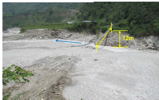
Plate 11: Disaster area around the suspension bridge at Karapani (The flood overtopped the left-bank river terrace due to the momentary river blockage.)
