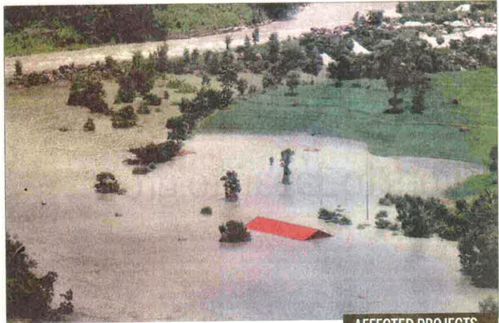
• A powerhouse of Sanima Sunkoshi project is submerged in the Sunkoshi River, on Saturday.
