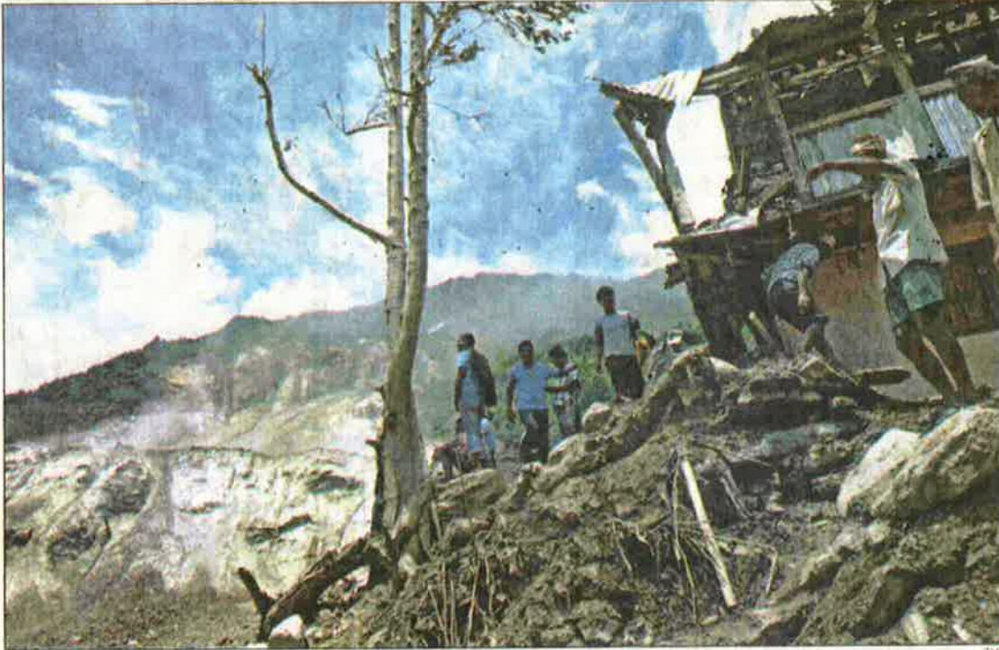
Locals at the site of a massive landslide in Jure of Ramche VDC, Sindhupalchowk, that blocked the Sunkoshi River on Saturday morning.
