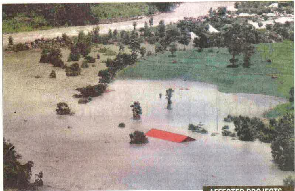
■ A powerhouse of Sanima Sunkoshi project is submerged in the Sunkoshi River, on Saturday.
