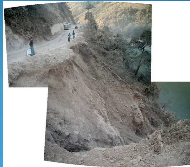
Broken retaining wall and road shoulder at Ch.33+000
