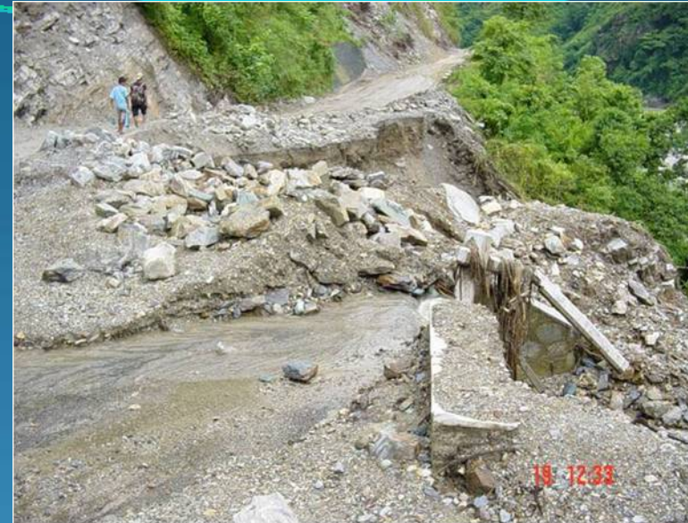
Broken retaining wall and road shoulder at Ch.33+000
