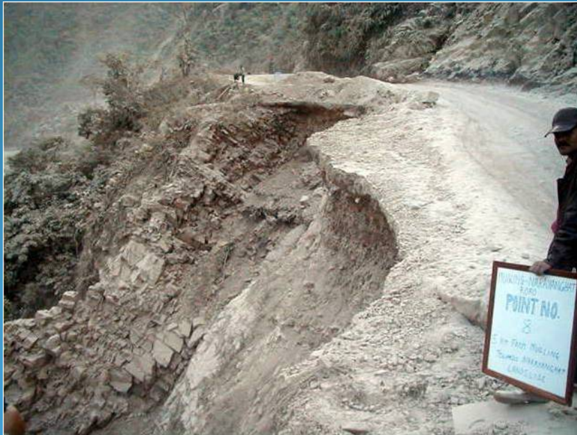
Broken retaining wall and road shoulder at Ch.33+000
