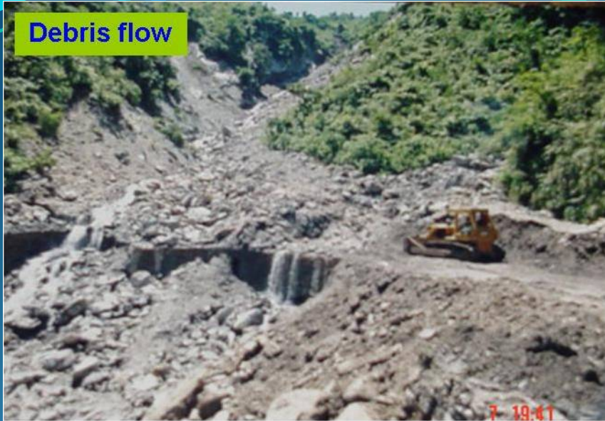
Broken retaining wall and road shoulder at Ch.33+000
