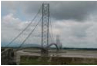
Dodhara Chandani 橋 (鋼製人道つり橋)
